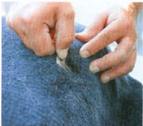
20 A single-edge razor was used to trim the carpeting away for the bolt-holes.
