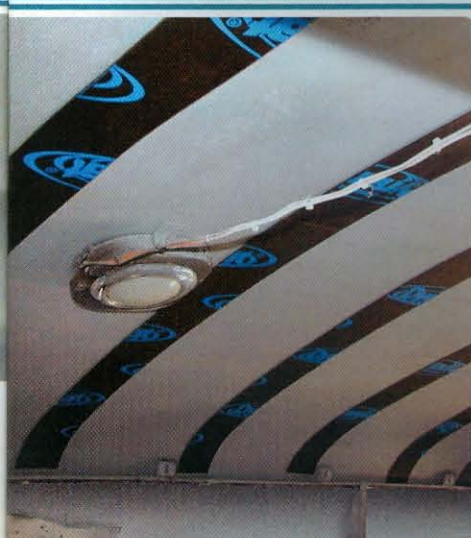
15) Here, those same strips are applied to the underside of the roof, a simple matter of peeling off the protective backing and sticking the adhesive-backed sound deadener in place.
