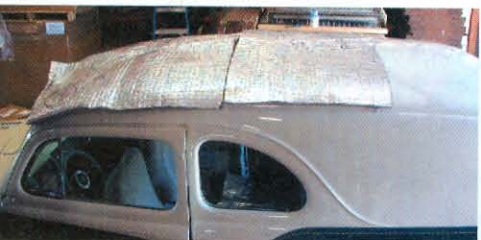
20) Next came the layout of the actual insulation (on top of the roof). Notice how it "pooches up" over the peak above the windshield. A kit piece for this position would have a wedge cut at that point to accommodate the shape.
