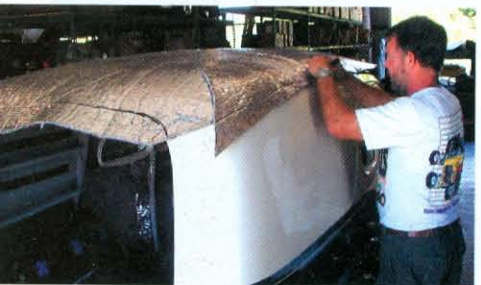
21) It took awhile for it to dawn on us why Cox was taking measurements, making patterns and marking cut lines on the outside of the car. Duh. It sure beats working upside-down underneath.
