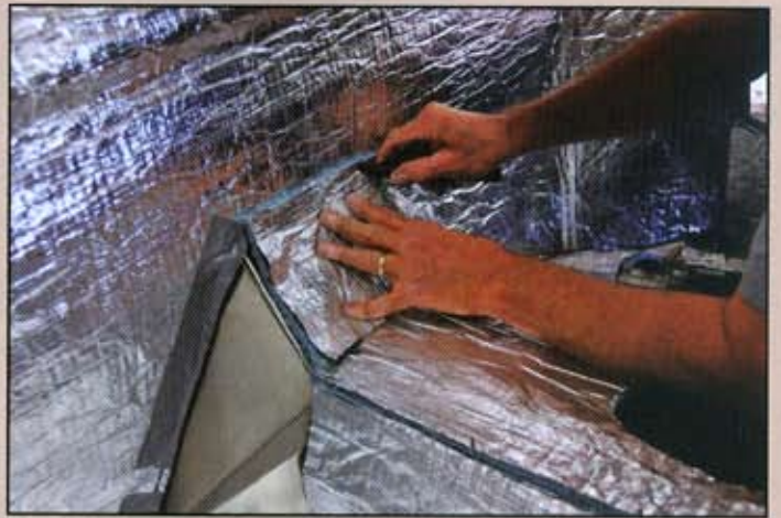
Note that foil tape should be used to seal the seams.
