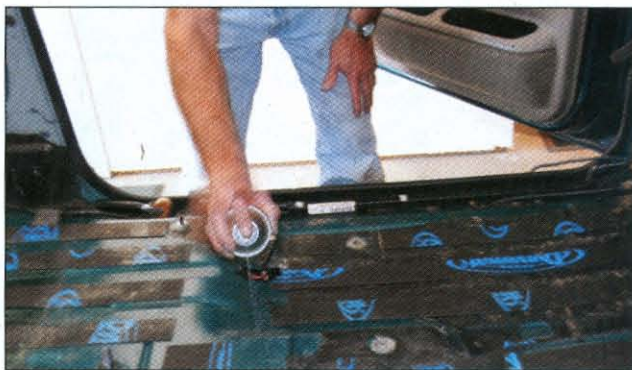
Apply the spray-on adhesive to the Dynamat strips.
